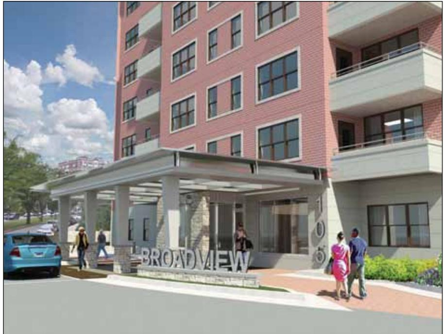
Exterior changes at the Broadview Apartments include replacement windows, removal of the HVAC units on the sides of the building, and new entrance canopies similar to the design depicted in this architect's rendering.
